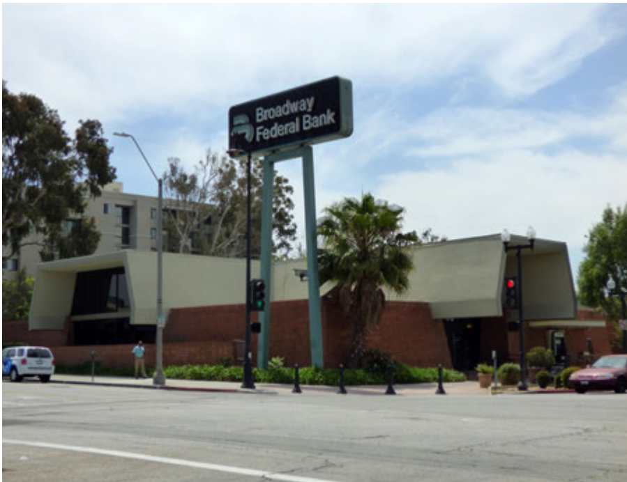
Former United Bank of California, 158-170 N. Market Street ( Southeast view ).
