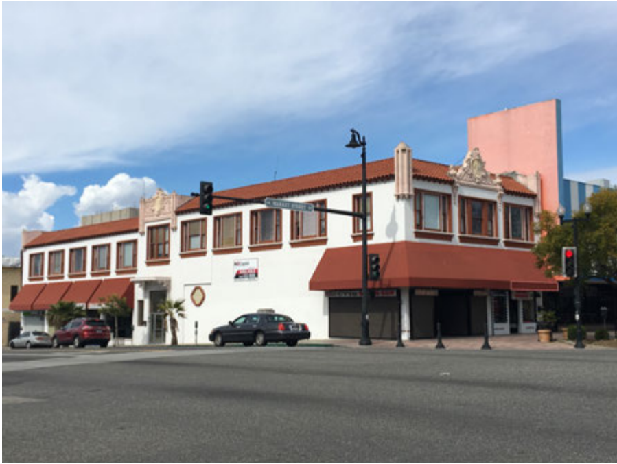
Professional Building, 149-155 S. Market Street/231-239 E. Manchester Boulevard (Northwest view).
