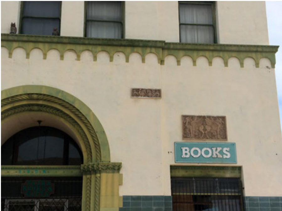
Former Bank of Inglewood, 100 N. Market Street/307 E. Queen Street ( East view, detail ).
