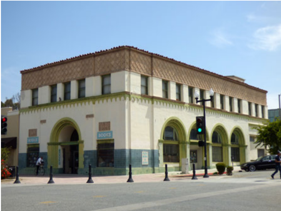
Former Bank of Inglewood, 100 N. Market Street/307 E. Queen Street ( Northeast view ).
