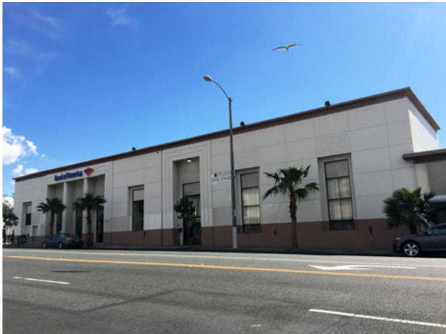
Bank of America, 320-330 E. Manchester Boulevard ( Southeast view ).
