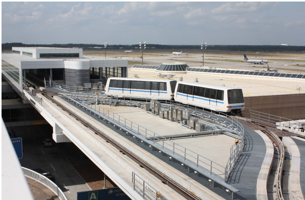
Figure 7-7: APM Double Crossover Example at IAH (Image Source: L+E)
