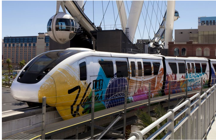
Figure 7-6: Monorail Emergency Walkway Example, Las Vegas Monorail (Image source: LAmag)
